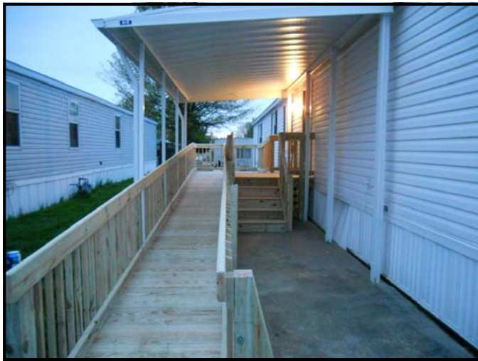
The finished ramp.
